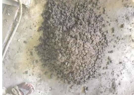
Fig.2.3: Mixing of Recycled aggregate concrete
