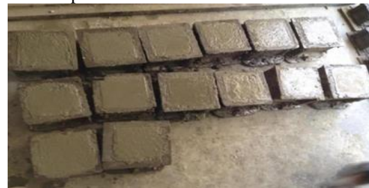
Fig.2.4: Mixing and casting of fresh concrete
