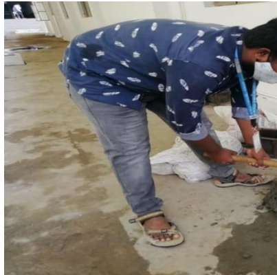
FIG-2.6. MIXING OF CONCRETE
