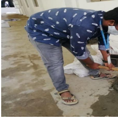
FIG-2.6. MIXING OF CONCRETE
